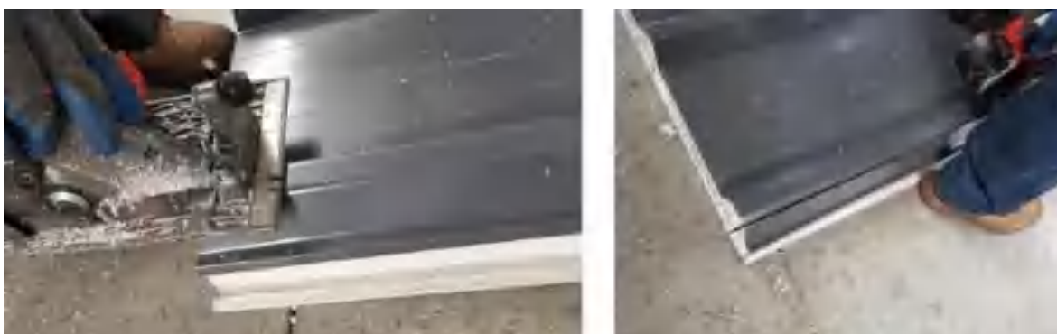
Figure 24 – End roof panels adjustment
