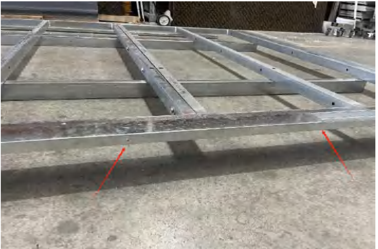
Using four rivets to secure the bottom piece to the U channel.
