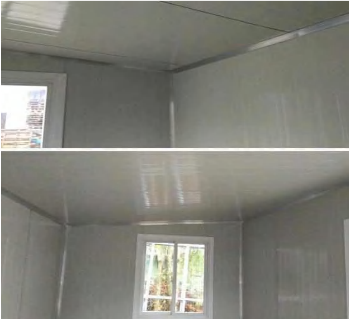
Interior aluminium angle trims
