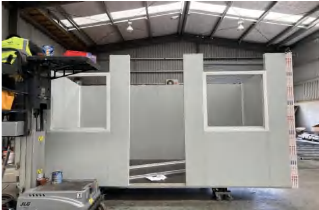
1. Assemble wall panels next to the PA door.
