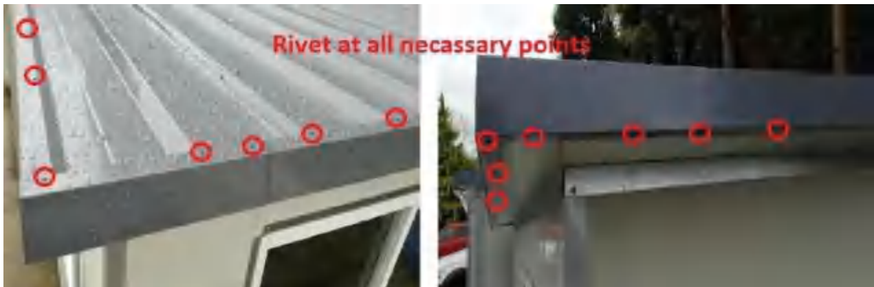
Roof flashing riveting
