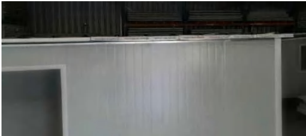
Roof panels positioned as straight as possible
