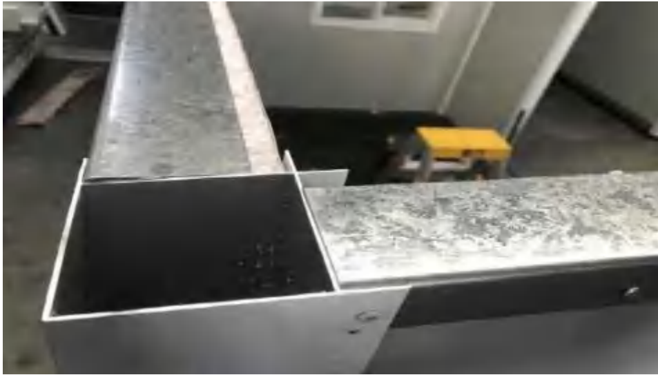
Aluminum pillar 'corner to corner' steel angle bar bracing
