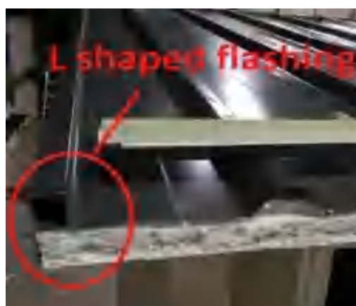
L shaped flashing
