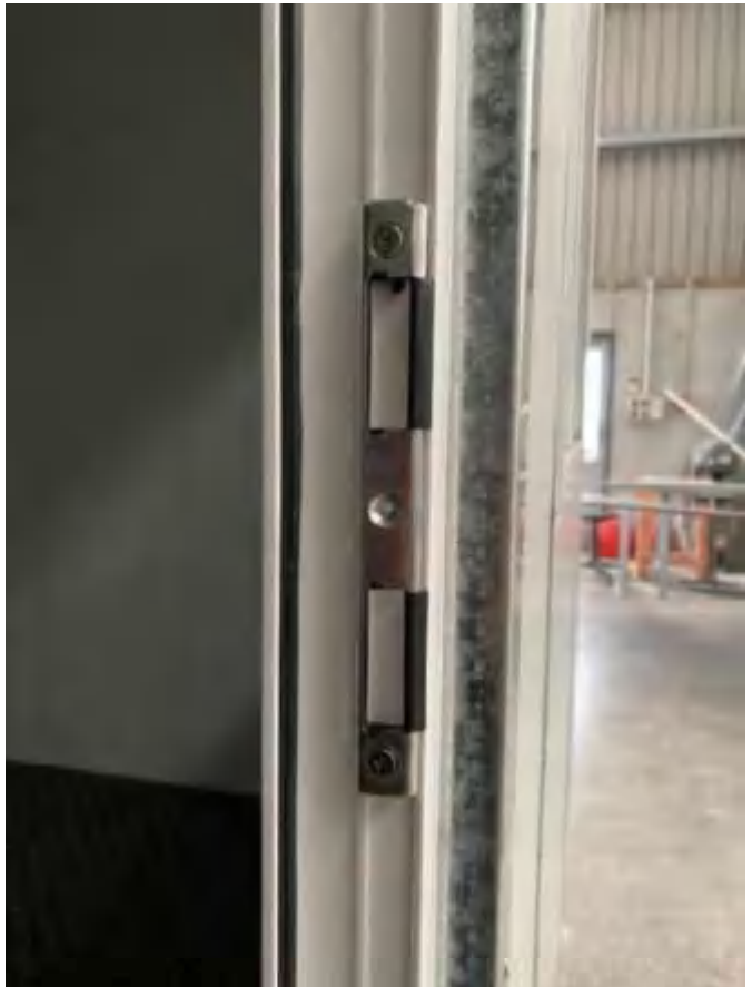
5. Attach door to the trim on three hinges
