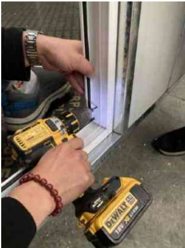
4.Adjusting the door trim to U channel frame
