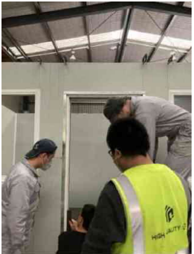
4.Adjusting the door trim to U channel frame
