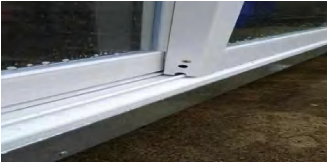
Slide door adjustment points
