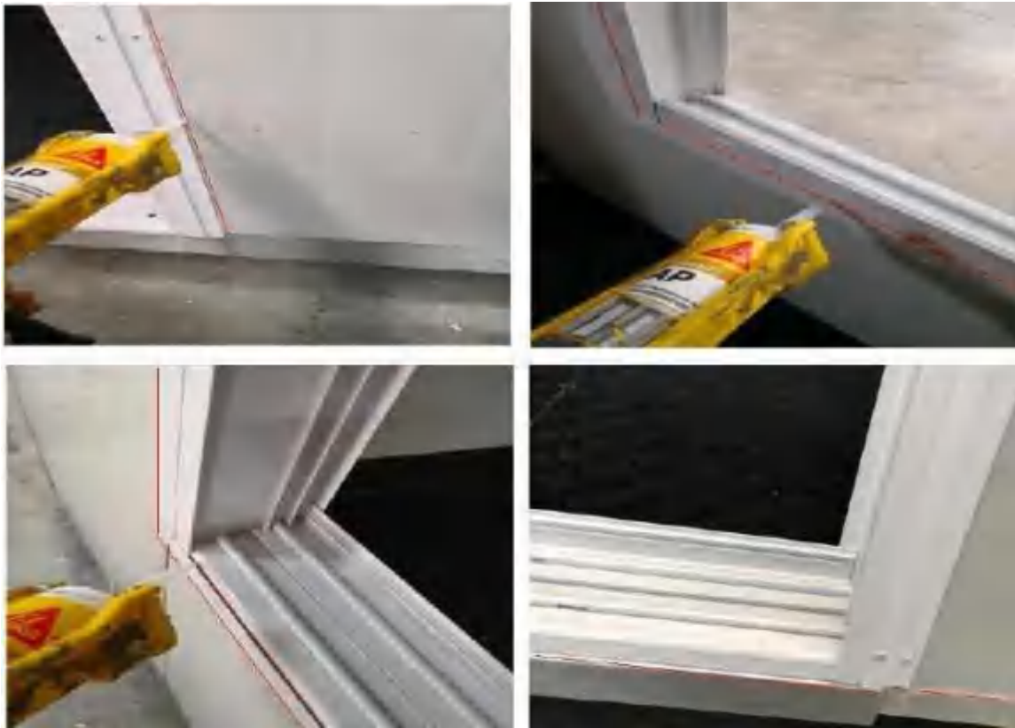
Weatherproof sealant / silicone application
