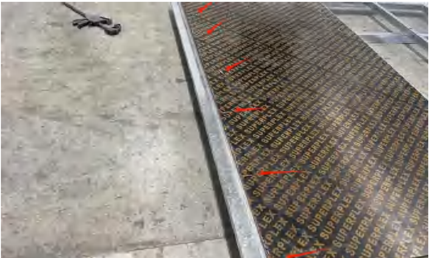
Using self-drilling/countsunk head screws supplied to attach plywood to steel frame.
