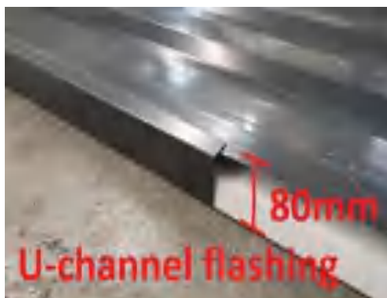
U Channel flashing
