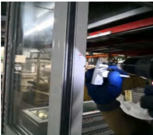
7. Use the 4.2mm drill bit to drill a hole
