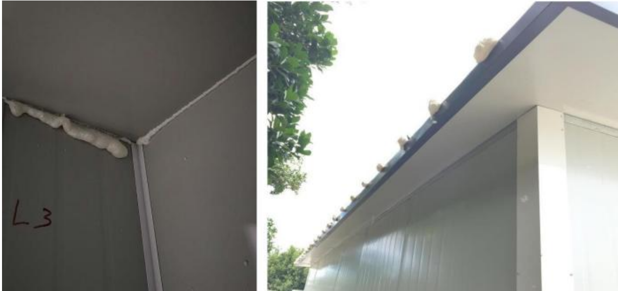
Figure 29 – Expanding foam application
