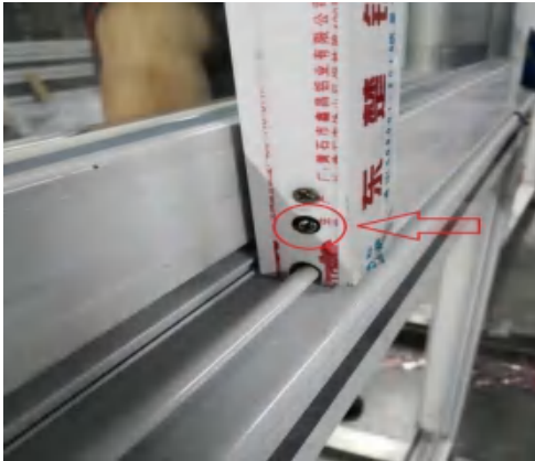
5.Use this screw to adjust the heightfor window lock Until the gap has been minimized
