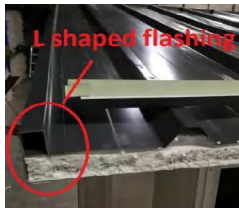
Figure 26 – L shaped flashing
