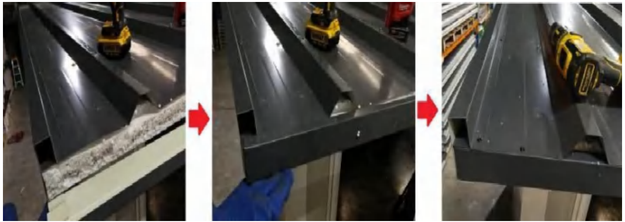
Figure 27 – 45mm double folded U-channel flashing
