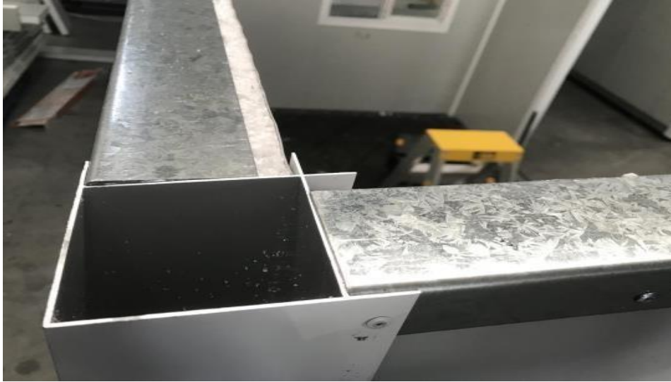
Figure 19 – Aluminum pillar ‘corner to corner’ steel angle bar bracing
