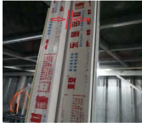
4. Check there is any gap between the Window with the Frame
