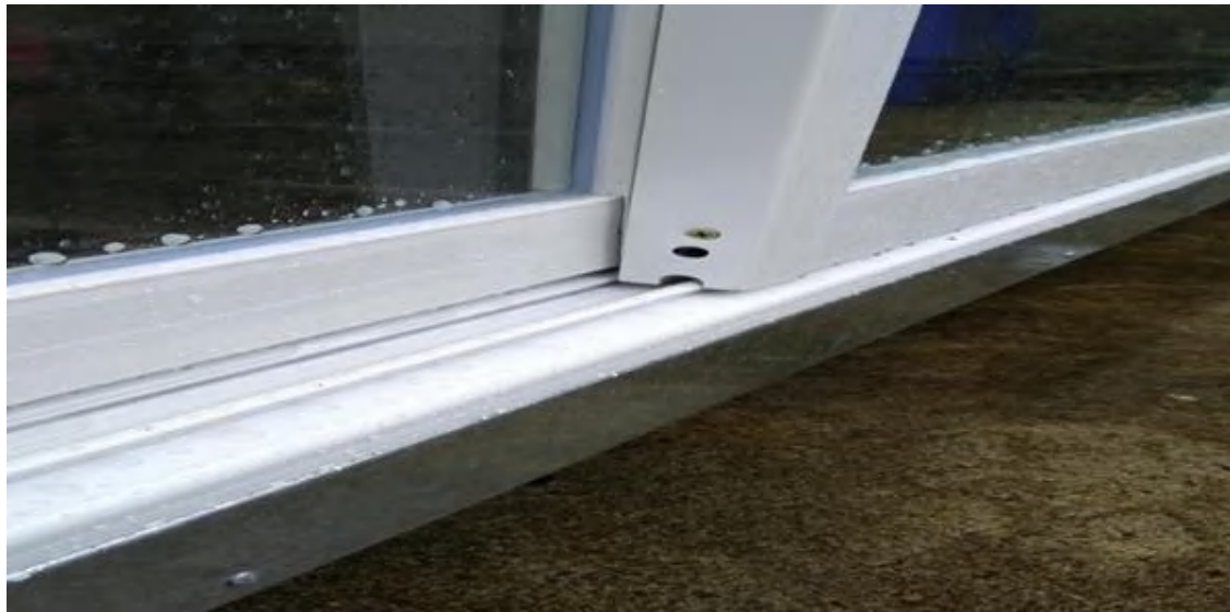
Figure 32– Slide door adjustment points
