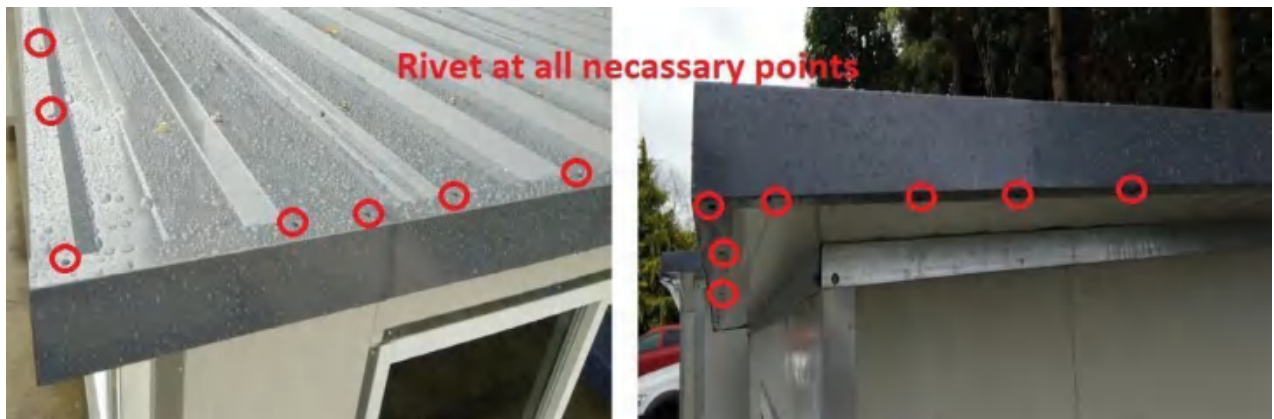
Figure 28 – Roof flashing riveting
