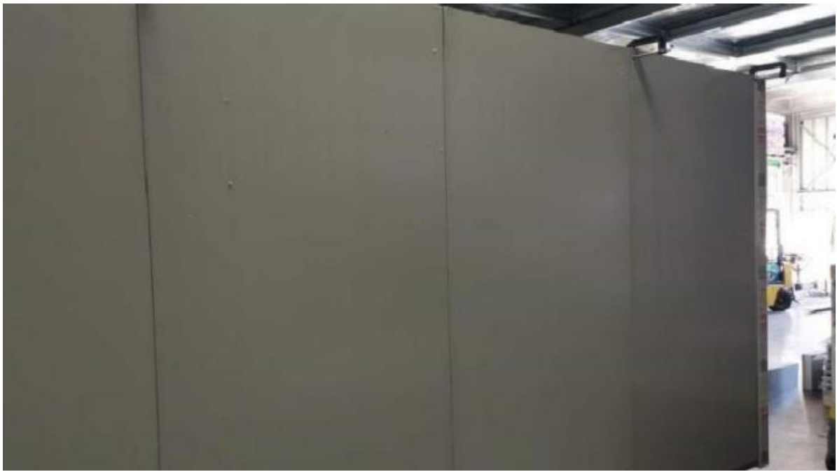
Figure 13 – Clamping wall panels
