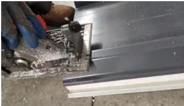
Figure 24 – End roof panels adjustment
