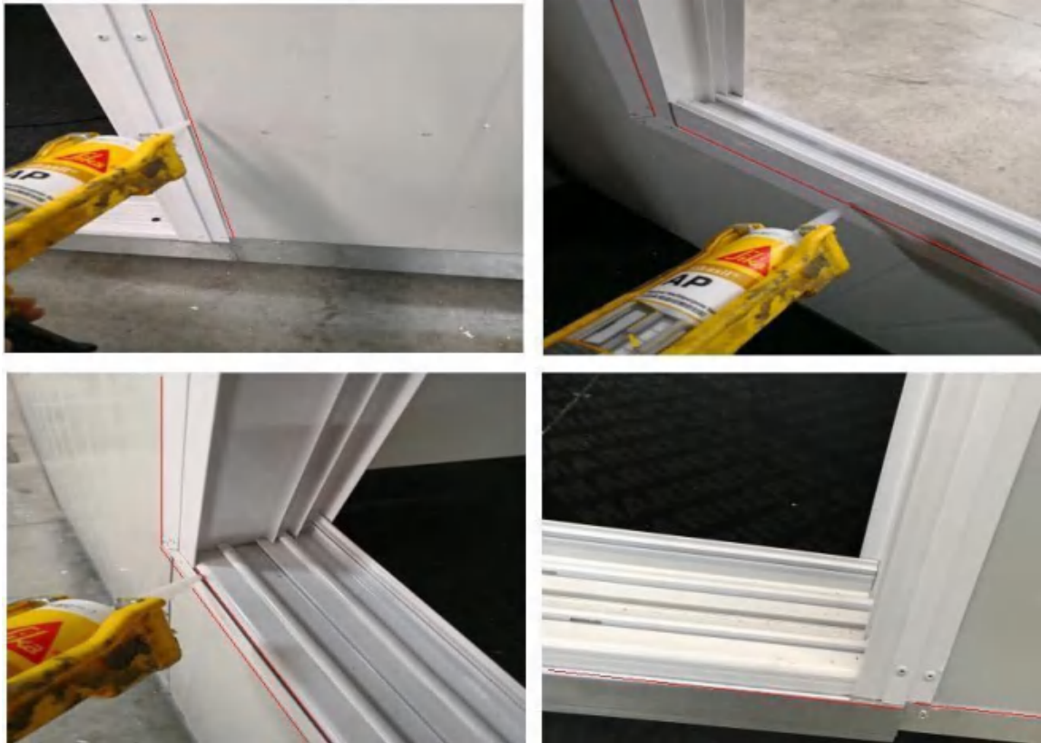
Figure 31 – Weatherproof sealant / silicone application
