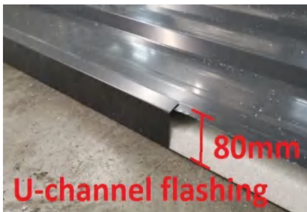
Figure 25 – U Channel flashing
