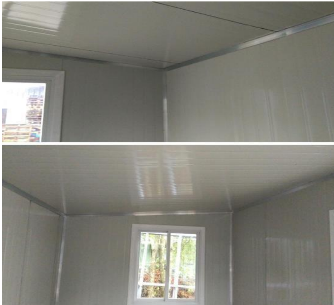
Figure 30 – Interior aluminium angle trims
