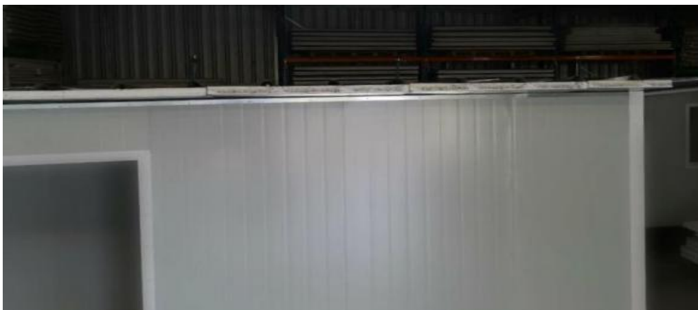
Figure 22 – Roof panels positioned as straight as possible
