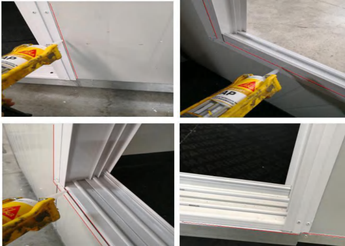
Figure 31 – Weatherproof sealant / silicone application
