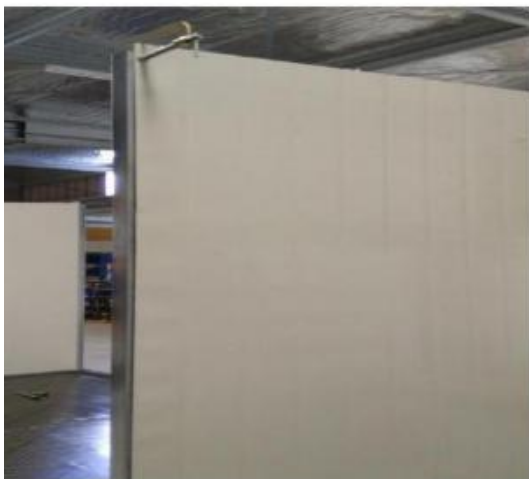
Figure 12 – Clamping corners
