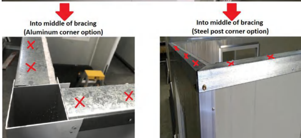
Figure 23 – Roofing panels attached to bracings
