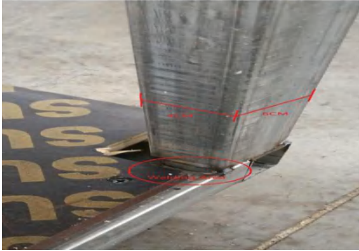
Figure 1 – Welded steel post
