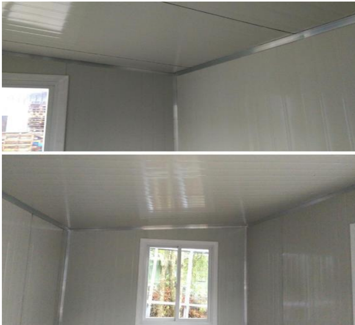
Figure 30 – Interior aluminium angle trims
