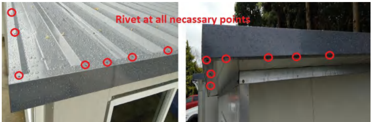
Figure 28 – Roof flashing riveting
