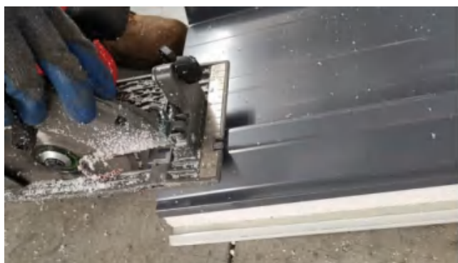
Figure 24 – End roof panels adjustment
