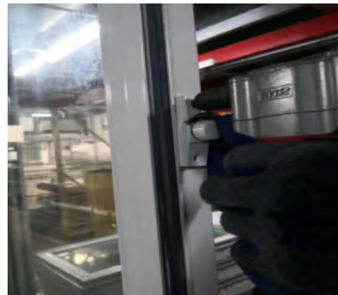
8. Use the white rivets to fix the lock to the window
