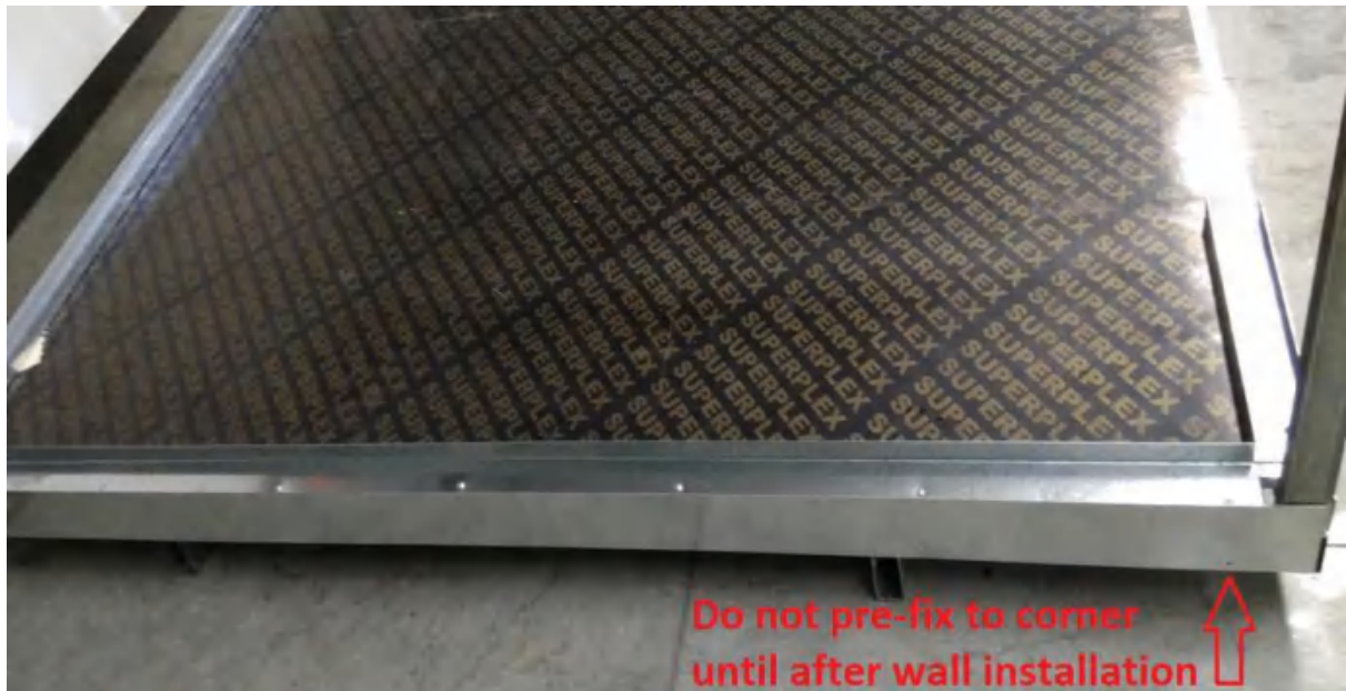
Figure 9 – Steel plates at corners (steel post option)
