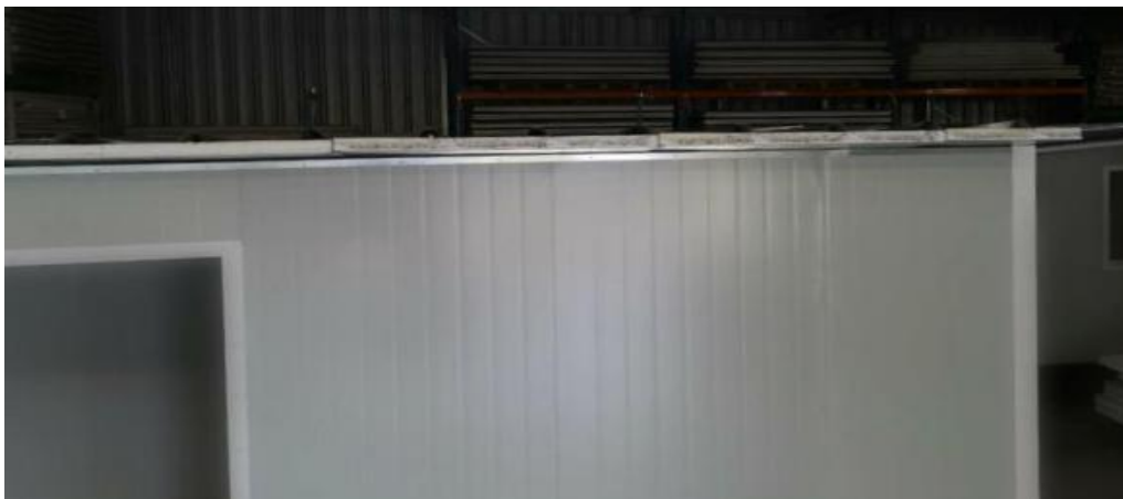
Figure 22 – Roof panels positioned as straight as possible
