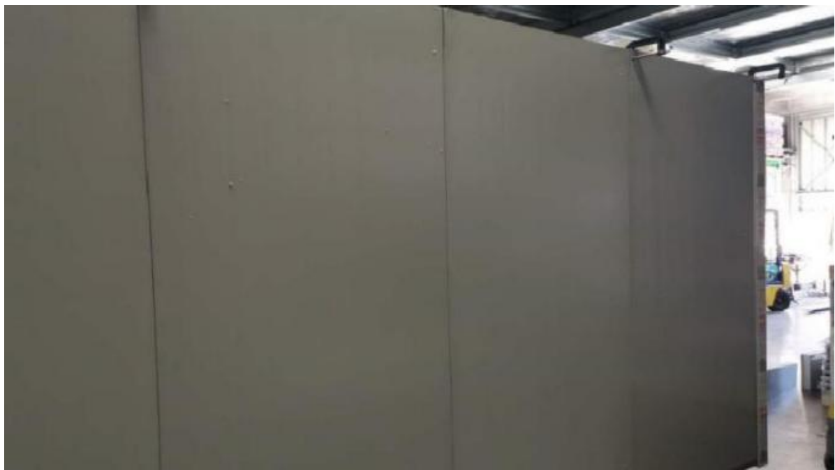
Figure 13 – Clamping wall panels
