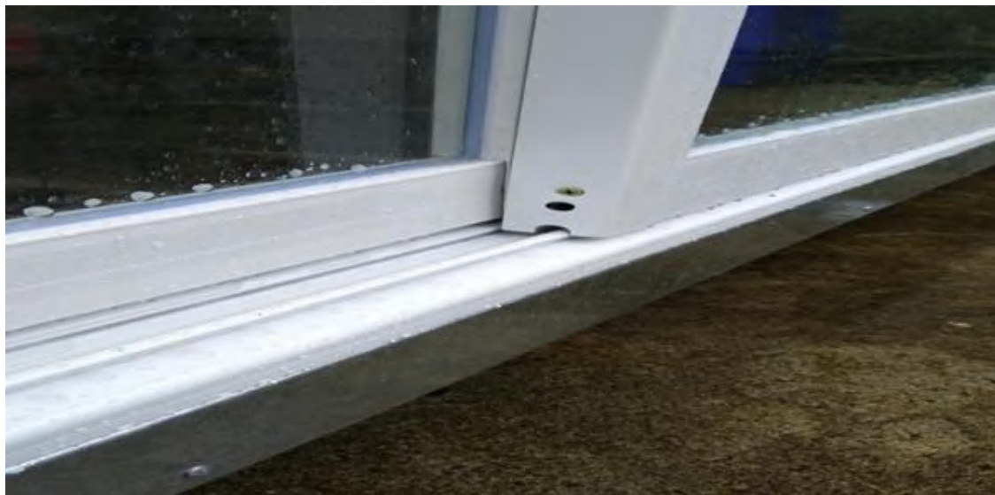
Figure 32– Slide door adjustment points
