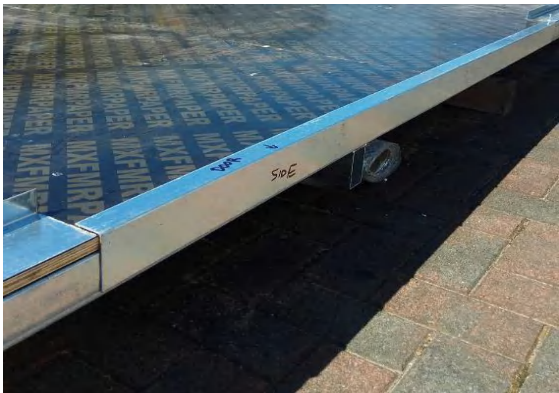
Figure 6 – Steel L-slots for slide door
