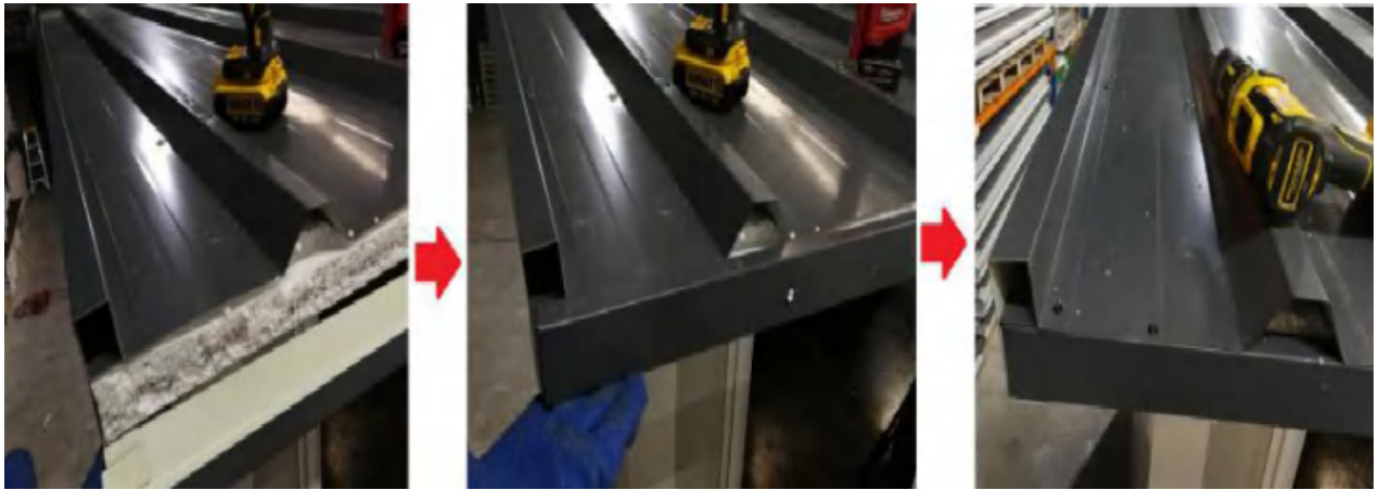
Figure 27 – 45mm double folded U-channel flashing
