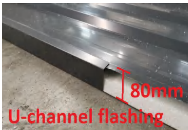
Figure 25 – U Channel flashing
