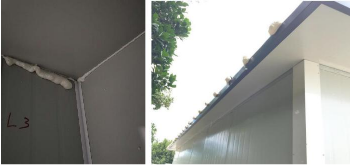
Figure 29 – Expanding foam application
