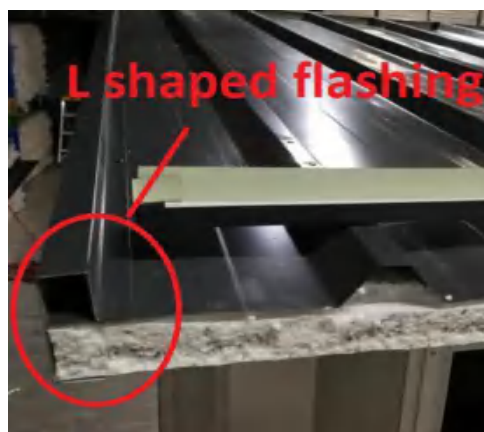
Figure 26 – L shaped flashing
