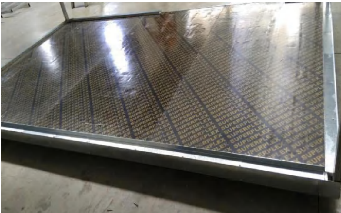
Figure 8 – Steel plates around perimeter
