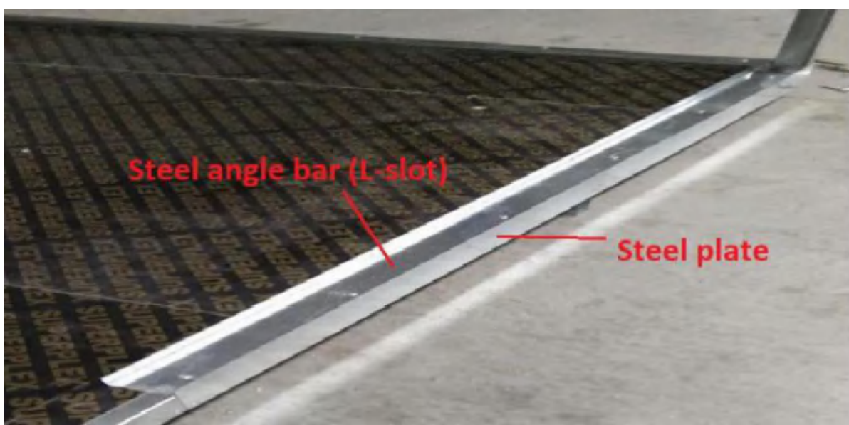
Figure 5 – Steel L-slots & plates
